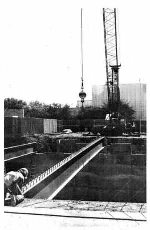
CONSTRUCTION of the underground addition to the SNLL Computing Center, now about 30 percent complete, is due to be finished by the summer of 1982. Ceiling beams, some 60 feet long, are here being installed. Wallace Webb & Son Construction Company of Hayward is project contractor.
